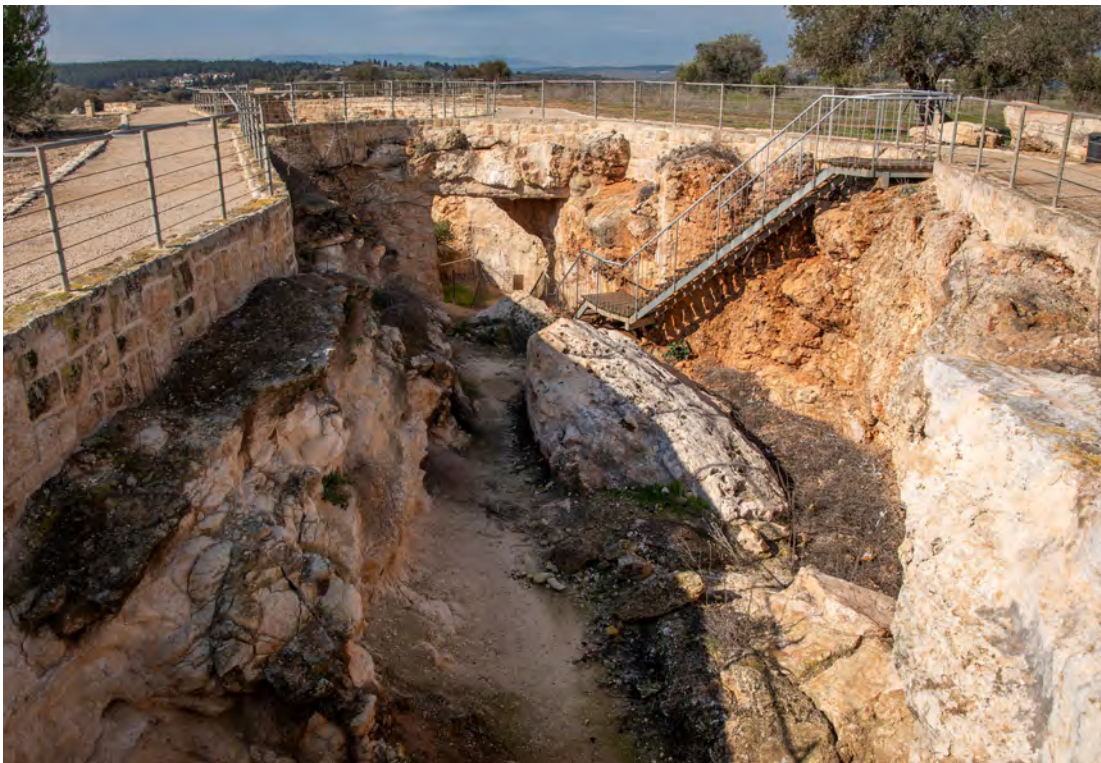
VIEW WEST: ROMAN-BUILT AQUEDUCTS FILLED SEPPHORIS'S IMPRESSIVE UNDERGROUND RESERVOIR THAT STORED WATER AND REGULATED ITS FLOW INTO THE CITY. THE RESERVOIR WAS REACHED THROUGH SIX VERTICAL SHAFTS.
